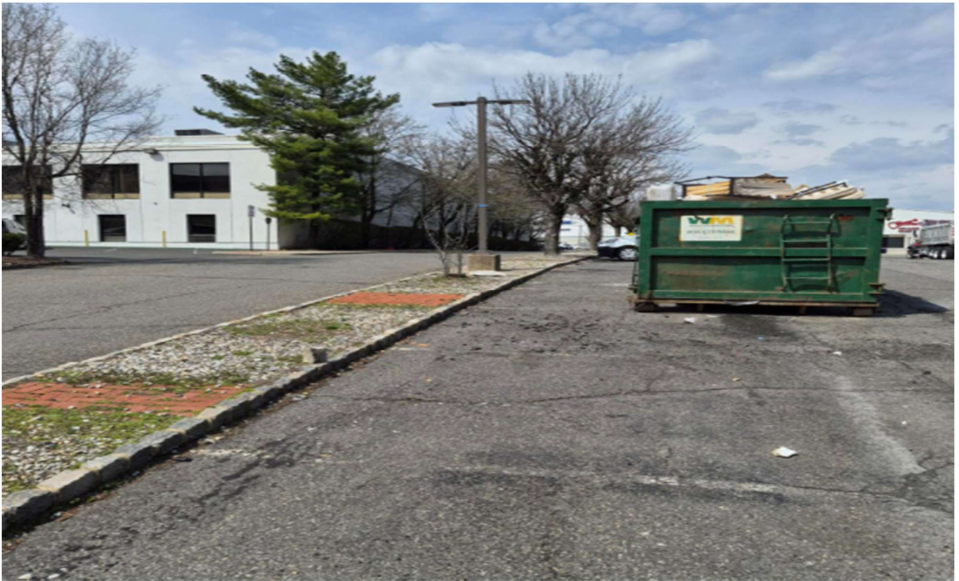
Photo 7: Parking lot facing west, showing parking and circulation-area conditions.
