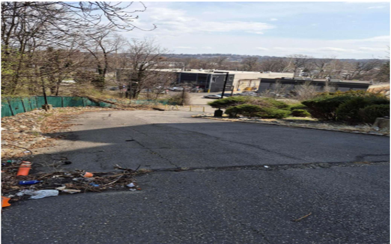
Photo 4: Southern driveway view facing east, showing driveway, pavement, and circulation conditions.
