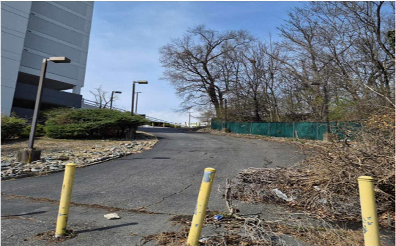
Photo 3: Southern driveway view facing west, showing driveway, circulation, and access conditions.
