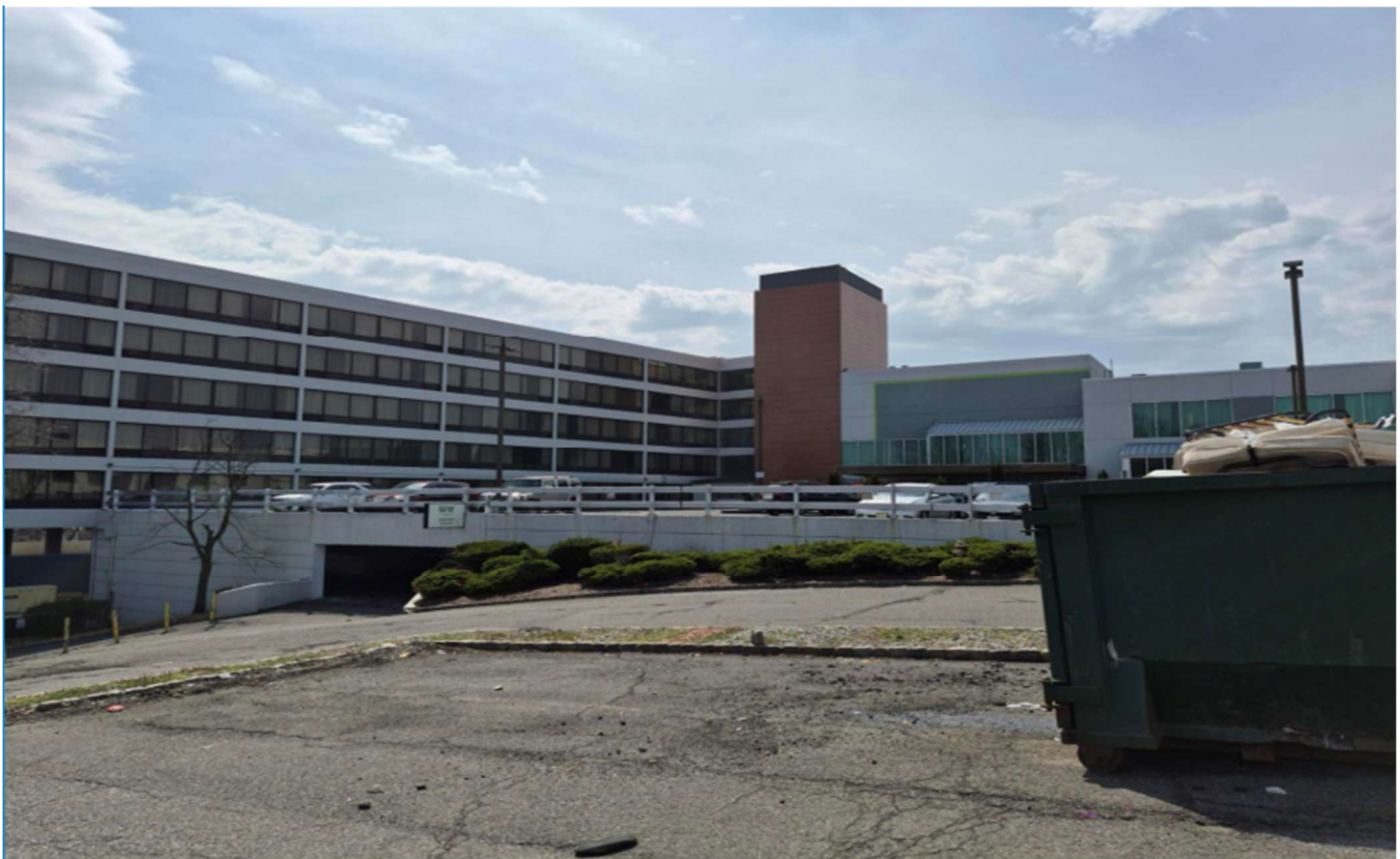
Photo 6: Parking lot and front entrance area, showing entrance-area pavement conditions and site circulation.
