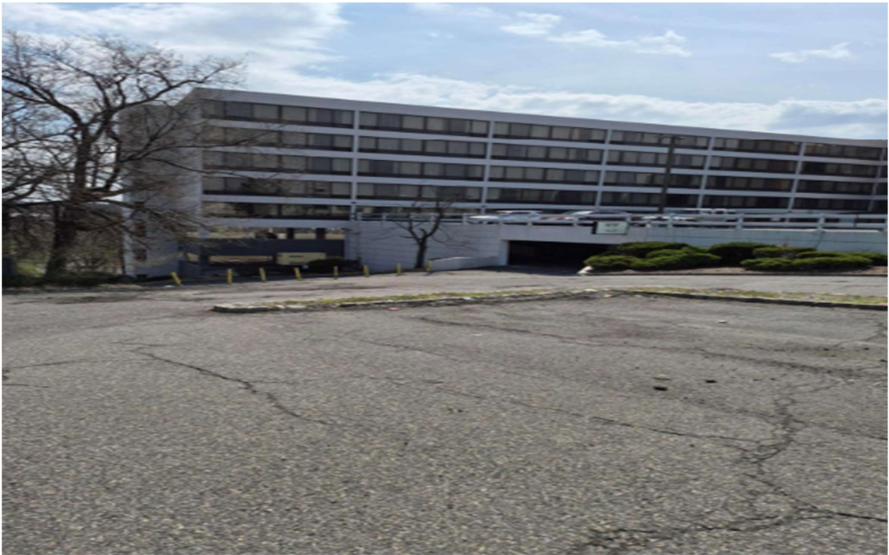
Photo 5: Parking lot facing east, showing parking-area pavement and surface conditions.
